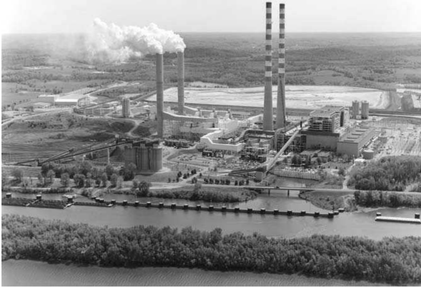
Figure 12.17 Aerial view of powerhouse and scrubber (courtesy of Tennessee Valley Authority).
